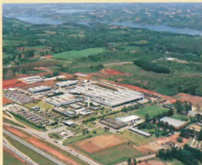
Fábrica/Fabrica/Plant: Curitiba, PR
